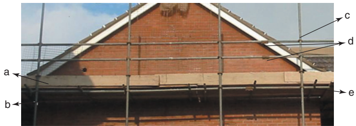
Figure 2.27 Typical scaffolding erection
