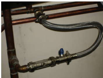
Figure 8.32 Typical approved filling loop
