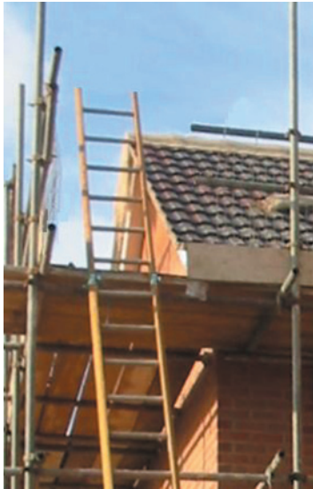
Figure 2.20 Safely lashed ladder
